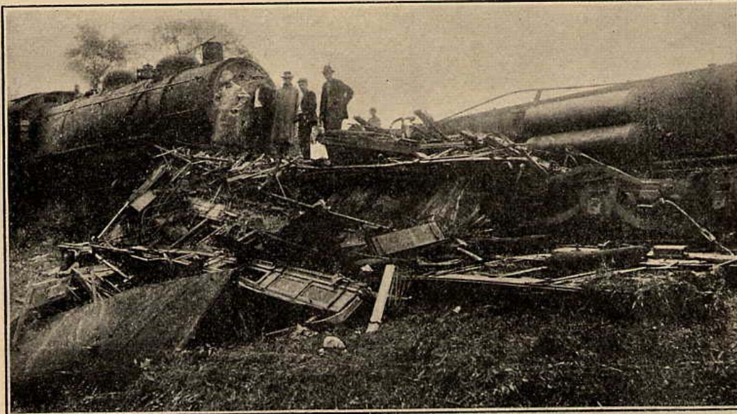
No. 1.—View showing demolished rear car, with the car next to the rear turned on its left side.
