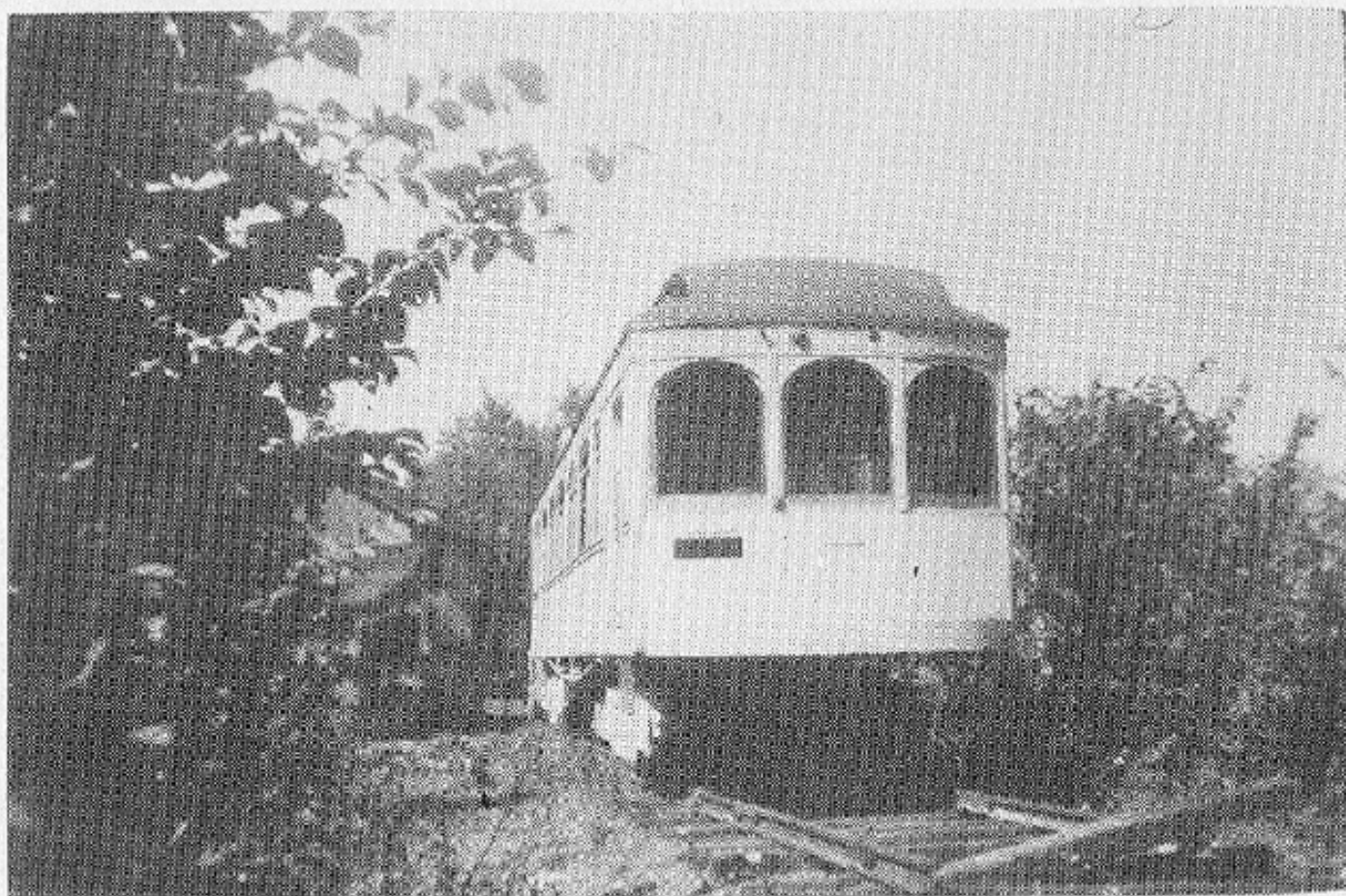
WINDOWS, ROOF, AND A PRIME COAT OF PAINT HAVE BEEN ADDED.
