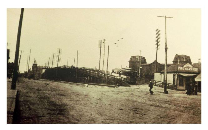
One of the Consolidated Street Railway Company's new electric street cars pulled an unpowered trailer across the High Street trestle. The temporary trestle bridged the seven steam railroad tracks that crossed High Street. Columbus Union Depot can be seen behind the man crossing High Street. Photo from the Ohio Historical Society Collection.
