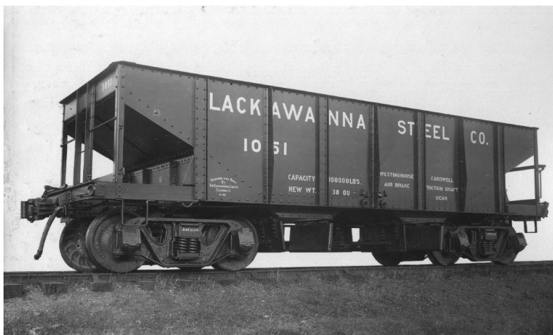
Ralston 50-ton twin hopper delivered in 1908. Note multiple drop-bottom discharge doors.
