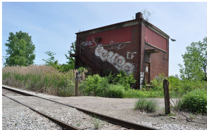
CW Tower, in repose. Photo by Ron Widman, 2014, from Columbus Railroads. CW controlled coal and other traffic moving to and from Grogan, Joyce Avenue and Pennor Yards, and on the CA&C track south to the Panhandle, High Street and the PRR Bradford and Miami Lines to the West.
