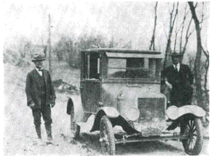
G. R. Stinchcomb, Subcontractor, R. N. Samson, General Superintendent in Car, E. H. Adams, Resident Engineer, Section No. 8.
