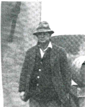
C. B. Randall, Concrete Foreman for the Walsh Construction Company.
