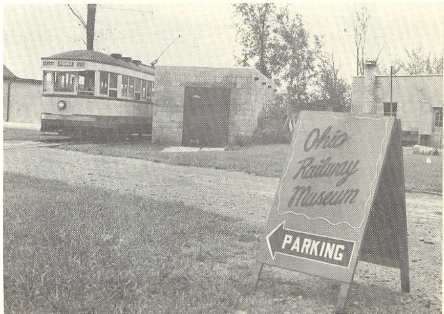
Car 3876 passing substation.
