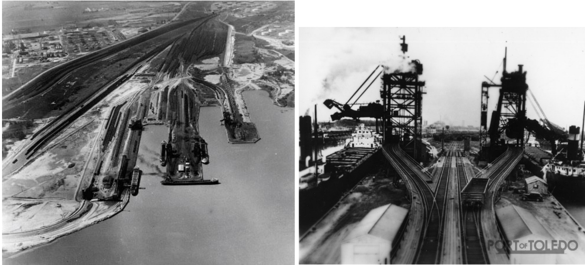
Left: Toledo's Lakefront Docks and adjoining rail yard facilities, 1940s. Right: Car dumper facilities, Toledo, 1940s. National Museum of the Great Lakes: https://nmgl.org/coal-dumpers-lakefront-dock/
