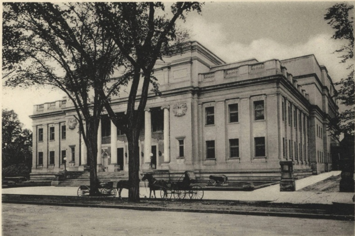
FRANKLIN COUNTY MEMORIAL HALL.
